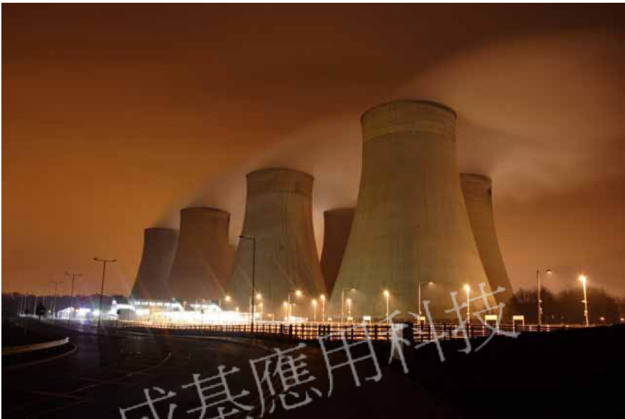
Figure 1. Natural Draft Wet Cooling Towers
